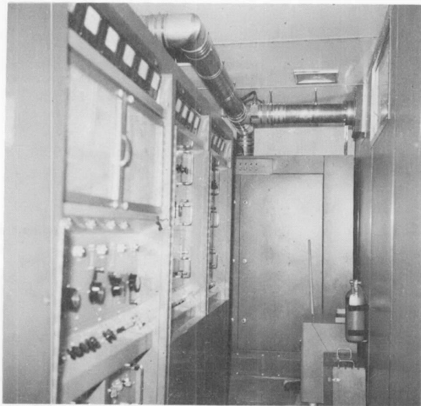
SYM-2006-TA1 Interior View
