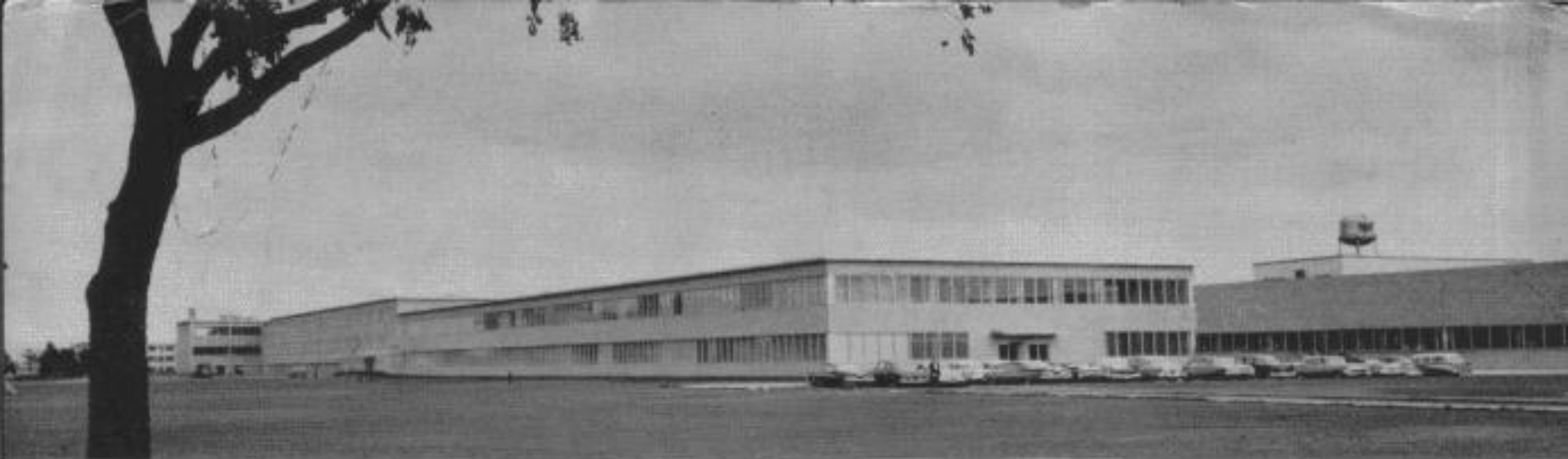
MODERN PLANT of Teletype Corporation is in suburban Skokie, Illinois.
