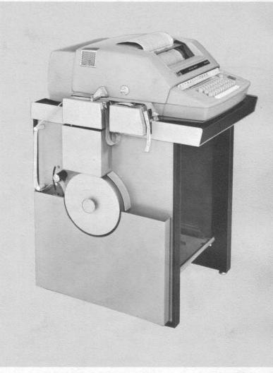
Teletypewriter Set AN/FGC-140() is an Automatic Data Set which is designed for continuous operation as peripheral equipment in a data processing system or as fixed station equipment in communication centers. The set combines a keyboard transmitter, medium speed receive page printer, high speed paper tape punch and reader, on a table. The console provides internal storage and automatic feeding for both roll and fanfoldpaper, and housing for interface and logic circuit boards, and dc power supply.
