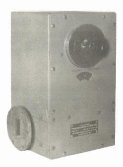
A portable, general purpose, self-contained and pre-calibrated frequency measuring cavity of the absorption type designed to measure the frequency of radio frequency signals in the range from 7050 to 8200 megacycles per second.
