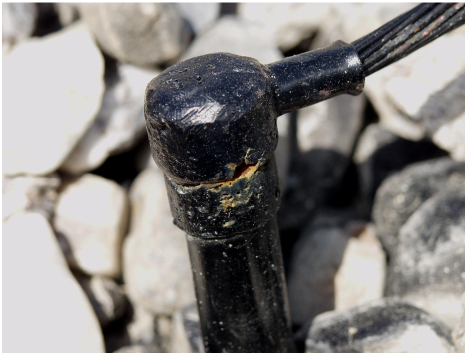
Figure 15 CADWELD ® on Antenna Counterpoise Wire
