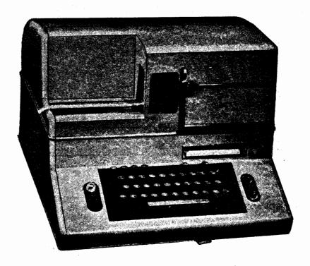
PERFORATOR-REPERFORATOR, TELETYPEWRITER TT-253/UG
