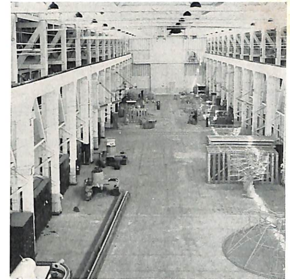
Antenna Shop, San Francisco Naval Shipyard. This spacious area is devoted entirely to the renovation of all types of radar antennas. A paint spray booth has been installed to handle the largest radar antennas. Two large cranes on tracks run the full length of the shop.
