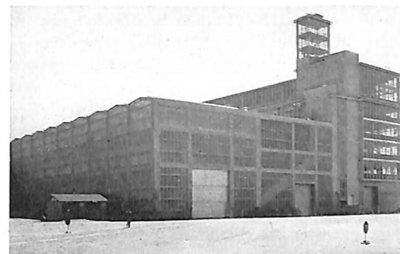
The home of electronics, Bldg 253, San Francisco Naval Shipyard. A complete set of radio and radar antennas are installed and operating seven and ten stories above the ground. An escalator takes personnel to their working areas and return. An elevator in the front and one at the rear take freight and passengers up and down six floors.
