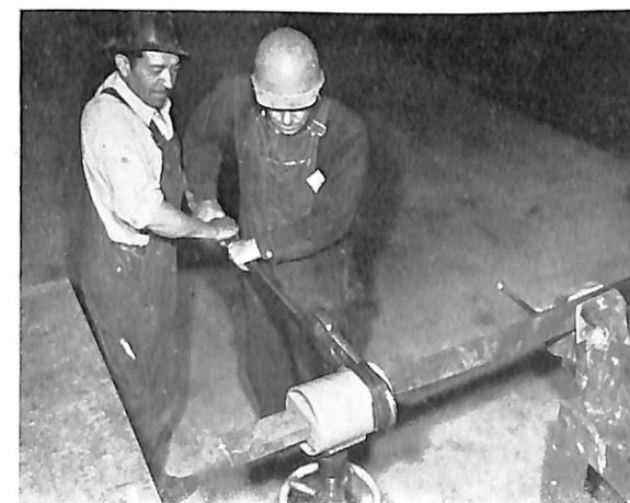
Shop 56 personnel twisting waveguide.
