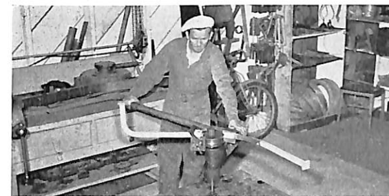
Bend being made by Shop 56 pipefitter.
