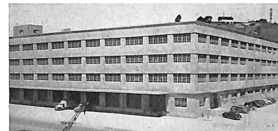
Electronics Supply Bldg. 813, San Francisco Naval Shipyard. Home of 40,000 electronic items.
