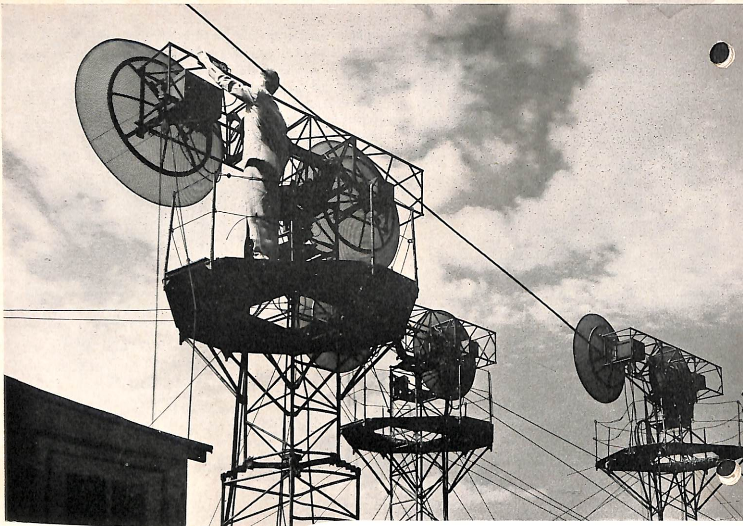
Rear view of three parabolic antennas on roof of the Telephone Building, New York City.
