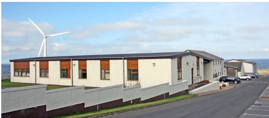
Figure 5: Forss Business and Technology Park office units. 9 September 2013.
