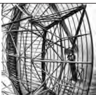
Texas Tower communication antenna
