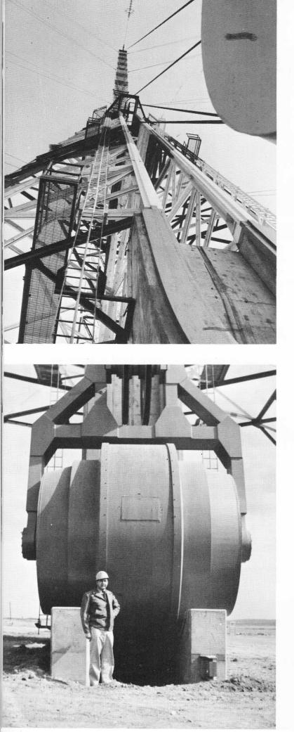
Each of Cutler's 26 sky-piercing towers pivots on a pointed base. Towers are supported by guy wires and adjoining rigid structures rigged with counterweights. Left-Counterweight track, main tower above.
